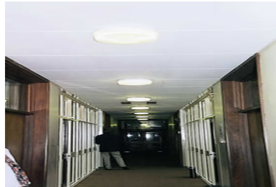
Suspended AIB ceiling tiles in a corridor
