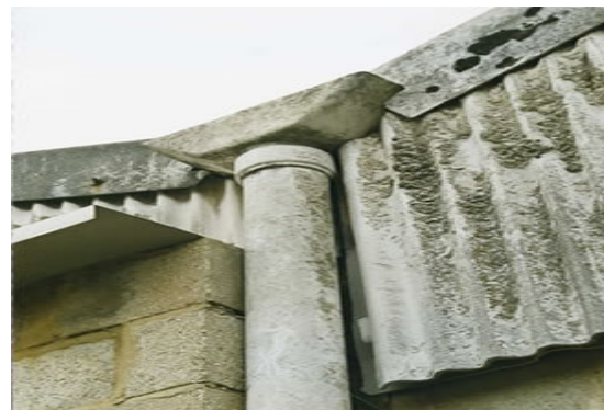
Asbestos cement downpipe, hopper and profile sheet
