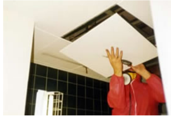
Careful handling of an AIB ceiling tile during removal
