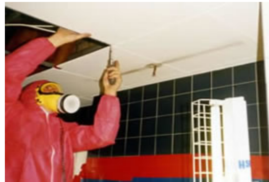
Unscrewing of an AIB ceiling tile
